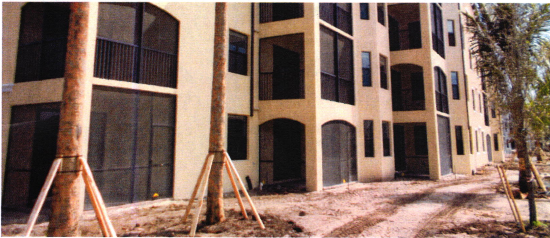
REAR VIEW (Picture taken 02/28/14)
