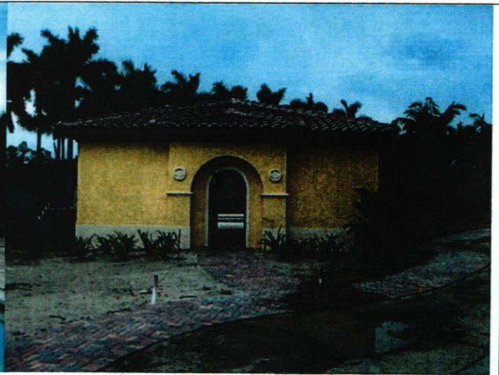
Rear of Building 12 July 2013
