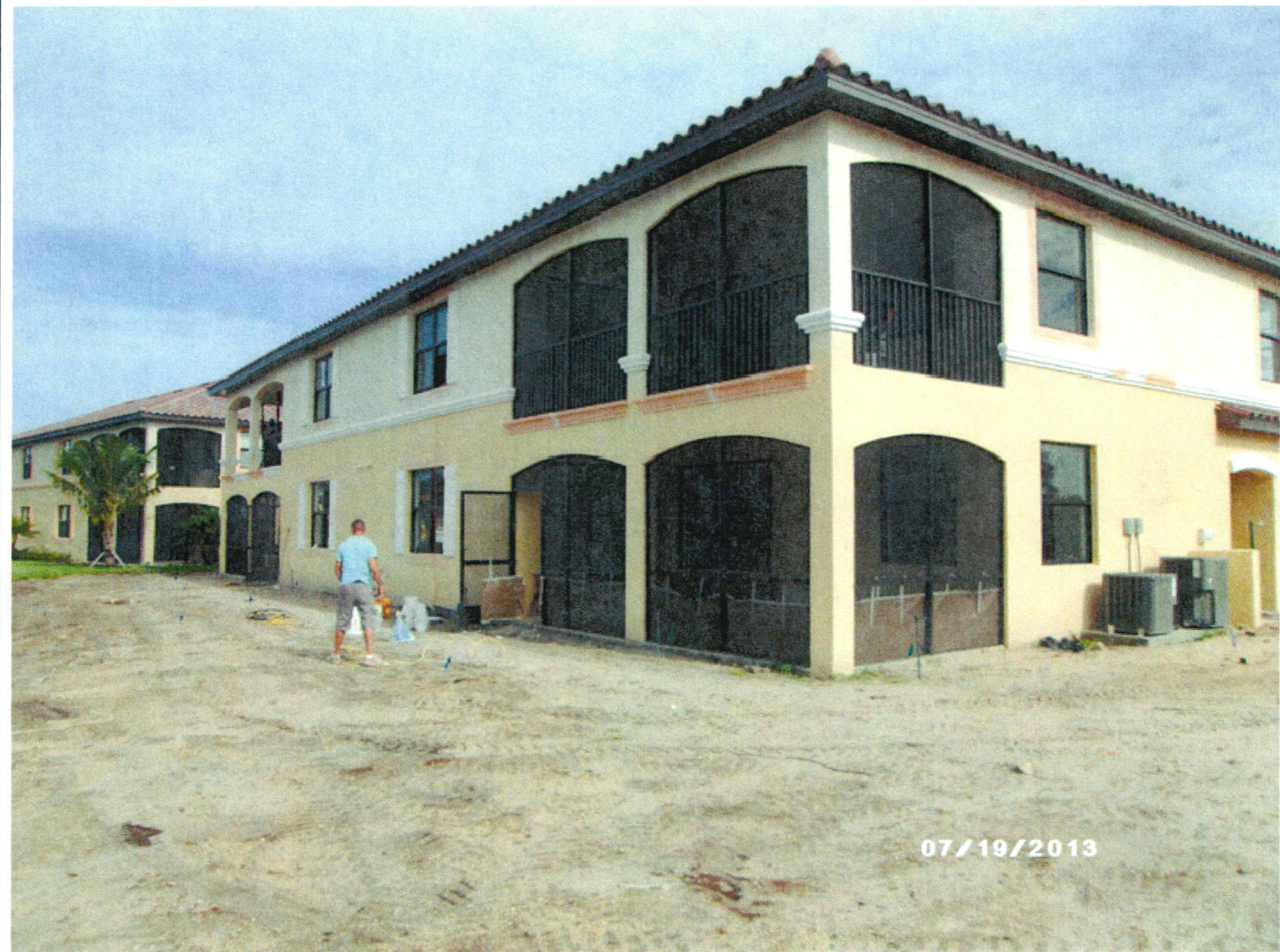
REAR VIEW (Picture taken 07/19/2013)
