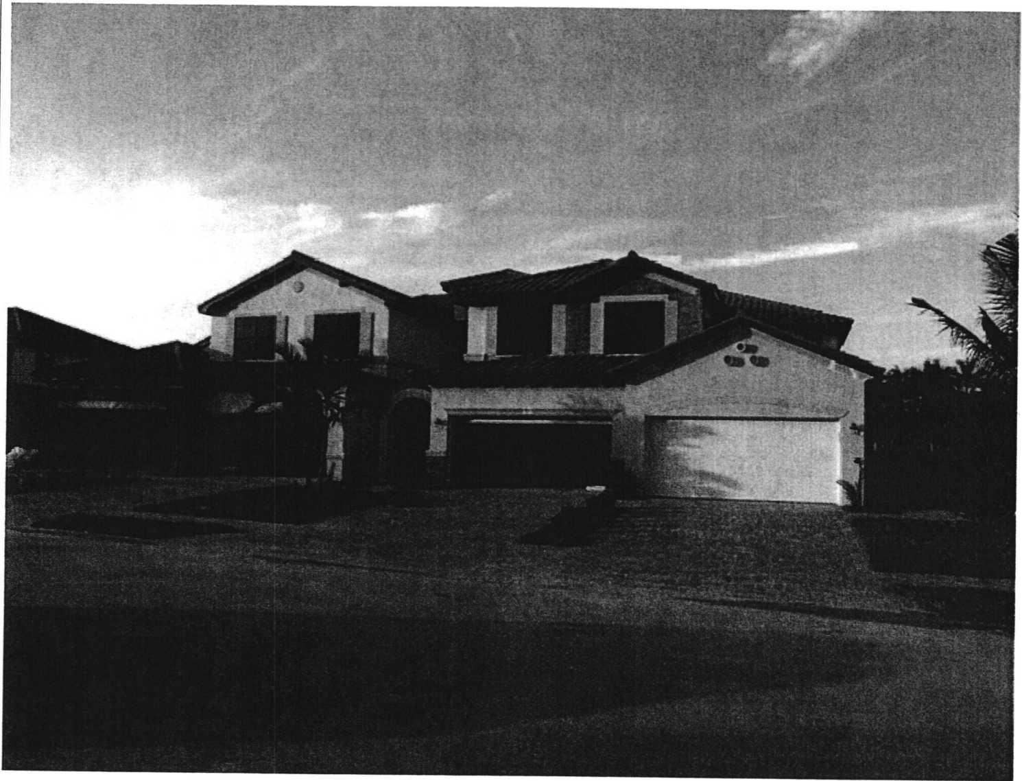
FRONT VIEW (PICTURE TAKEN 11/06/2013)
