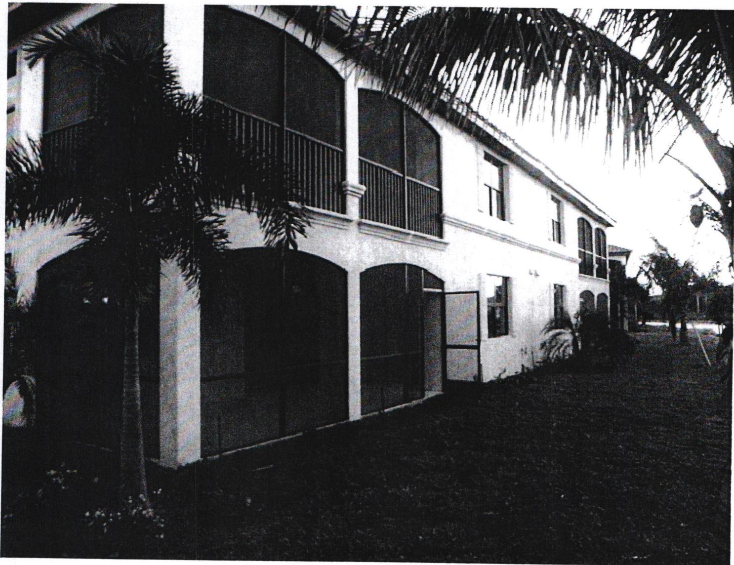
REAR VIEW (Picture taken 11/06/2013)
